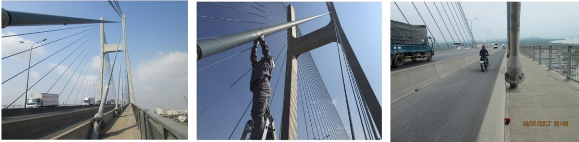
Fig. S1 Photos of Phu My cable-stayed bridge
