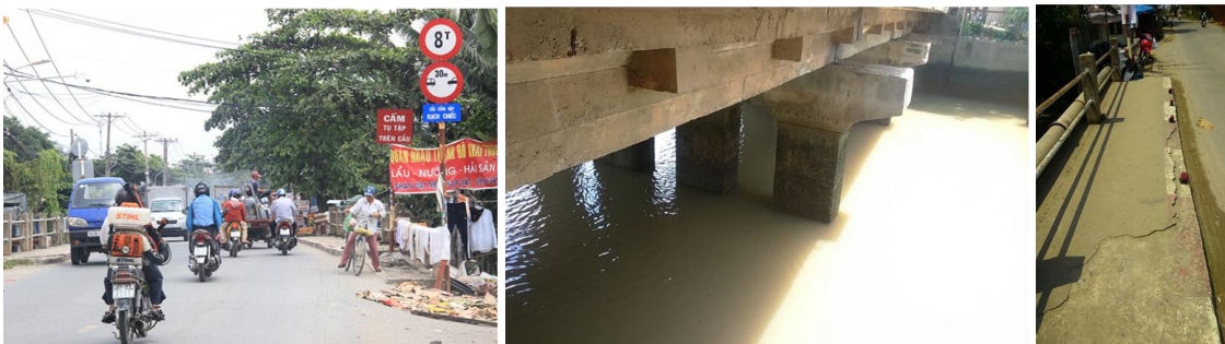
Fig. S4 Photos of Cong Dap Rach Chiec bridge
