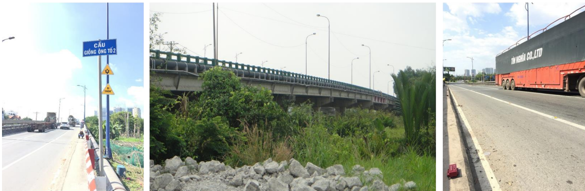
Fig. S2 Photos of Giong Ong To 2 bridge
