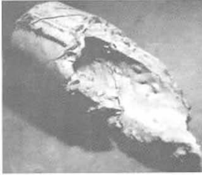
Fig.6 Failure of the inside concrete
