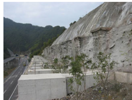
Fig. 6 Double-row stabilizing piles in Hongyan landslide
