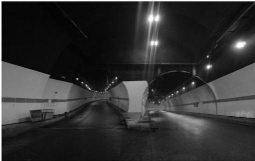
Fig. 12 Bifurcation surface of the tunnel
