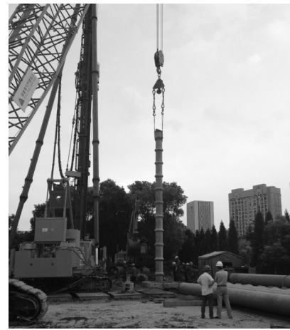
Fig. 5 Test pile installation
