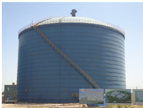
Fig. 1 A practical ground-supported circular steel silo
