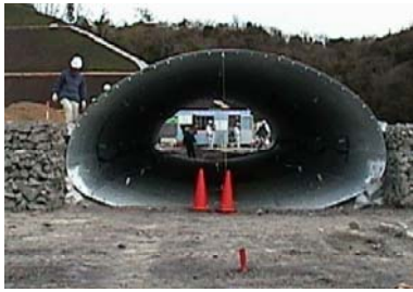
Fig.1 Corrugated steel culvert
