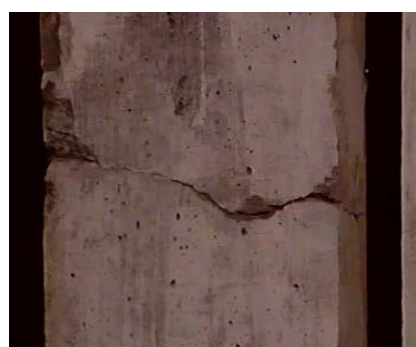
Fig.5 Crack after an unstable failure
