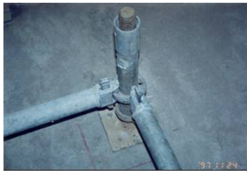
Fig.4 Jack base of a system scaffold
