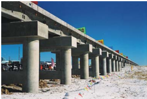
Fig. 1 A dry bridge on the Qinghai-Tibet Railway
