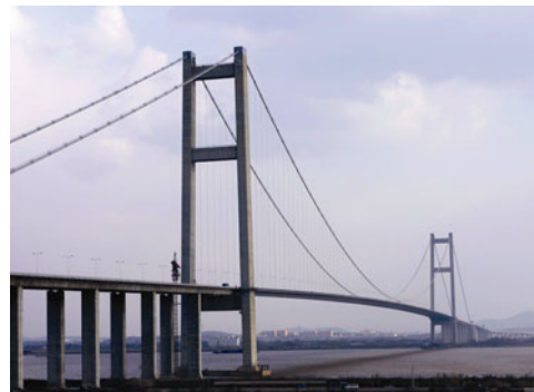
Fig. 1 View of the Runyang Suspension Bridge
