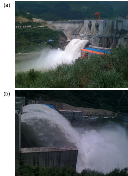
Fig. 1 Flood discharge with ski-jump flow of Wudu dam spillway in China (a) Elevation view; (b) Side view
